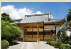
Renovation of the main hall
