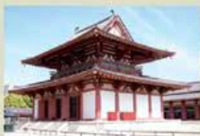
New main hall construction
